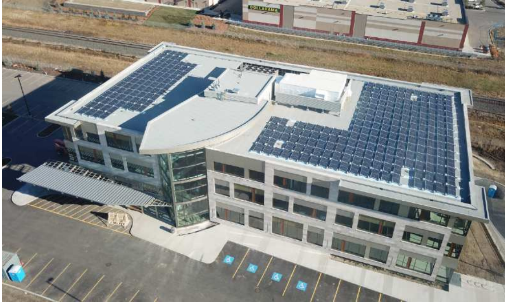
Figure 5.4: Solar Panels on a building (“BIPV and Architectural Solar Panel Applications”)
