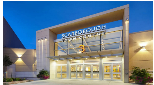
Figure 2.1: Scarborough Town Centre (Lamelza, 2018)
